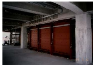
Viscous seismic damping wall
